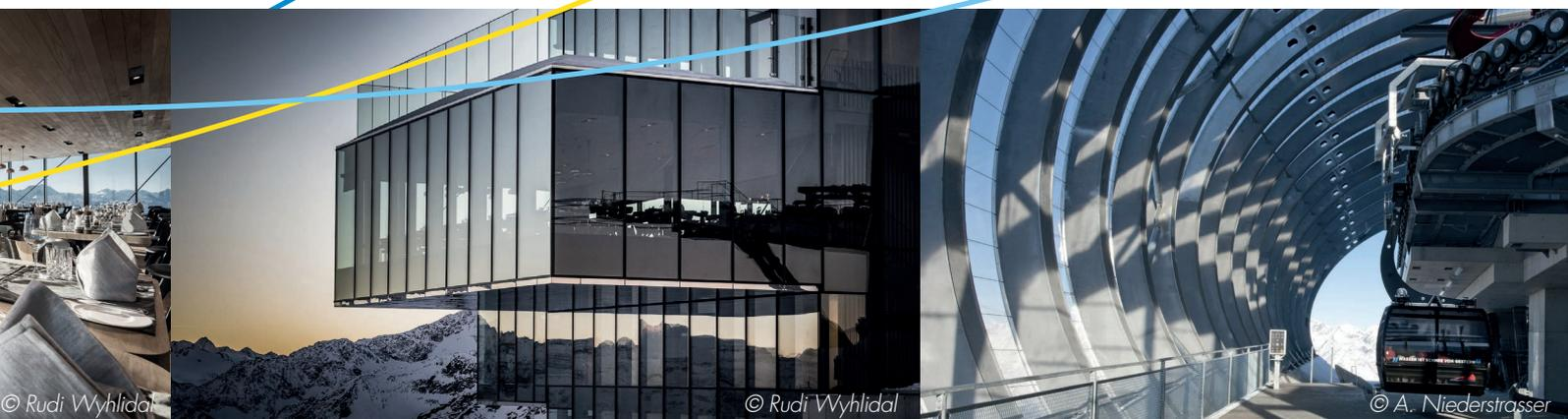
with rear ventilation was installed. SAUTER was tasked with regulating the entire system using a modern building automation system. This means that ice Q is cosy inside while the temperature of the restaurant's extract air never exceeds 5°C.
